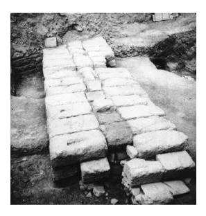
Figure 17 (above). Curtain wall at Dipylou 11 (Th8). Lower course of poros headers with anathyrosis; upper courses of conglomerate blocks. Elevation drawings of the wall, from the north (above) and from the south (below). Alexandri 1969, p. 44, fig. 14
