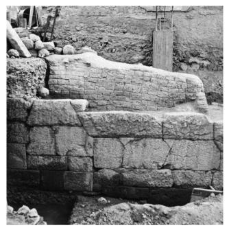
height of 0.70–1.04 m in two courses. 98 New sections in this form might have been constructed following the destruction or disintegration of the previous fortification.
