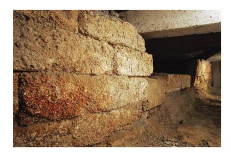
Figure 33. Themistoklean course, southern curtain wall at Dipylou 5–7–9 (Th9); view from the southwest. Reused poros block (center); limestone blocks on poros stretchers (at rear); conglomerate stretchers (foreground). Photo A. M. Theocharaki
