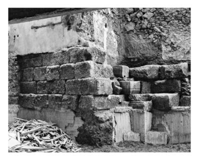
Figure 29. Hellenistic curtain wall of all-stone construction, Erysichthonos 15 (Th109). Note reused material in the core. Photo G. Hellner, courtesy Deutsches Archäologisches Institut (neg. D-DAI-ATH-Athen Bauten 669)
