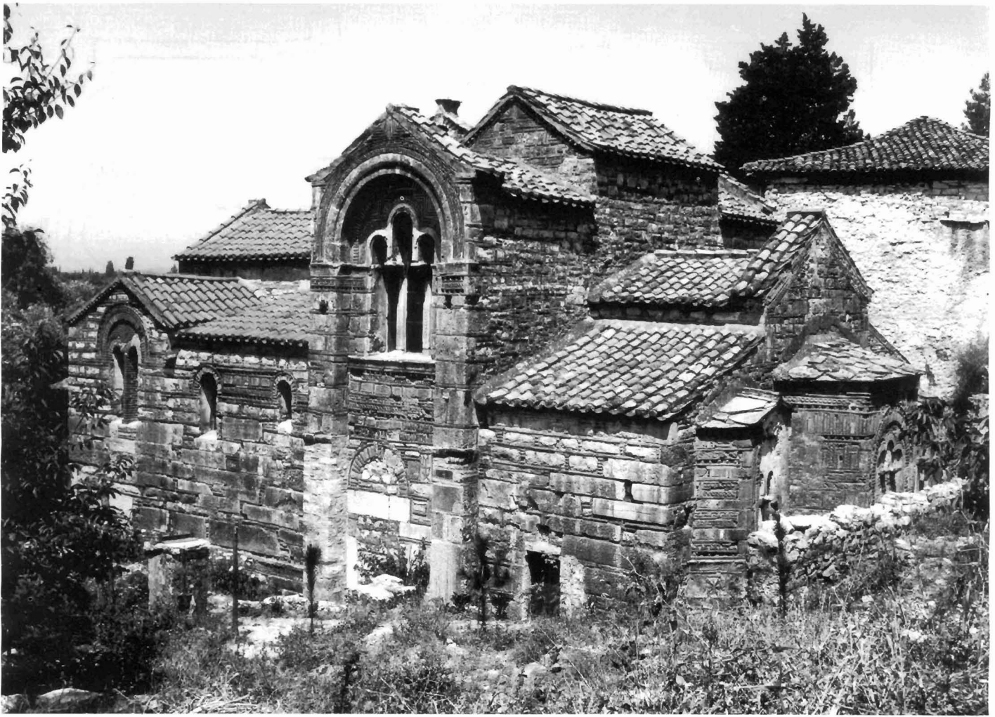
Fig. 3 Arta, Kato Panagia. Exterior from the southeast
