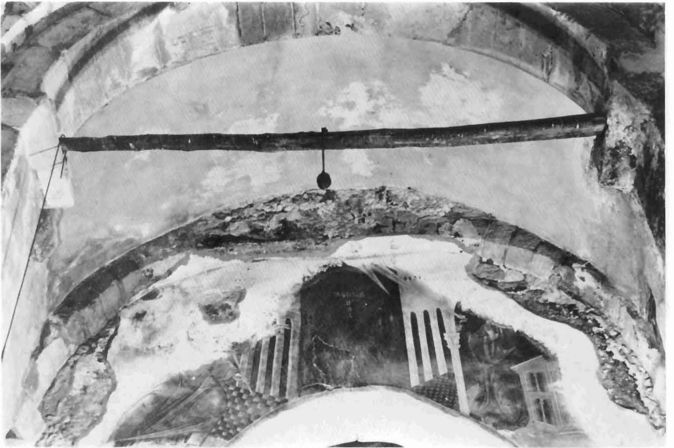
36. Vaulting, East End, and Bema
