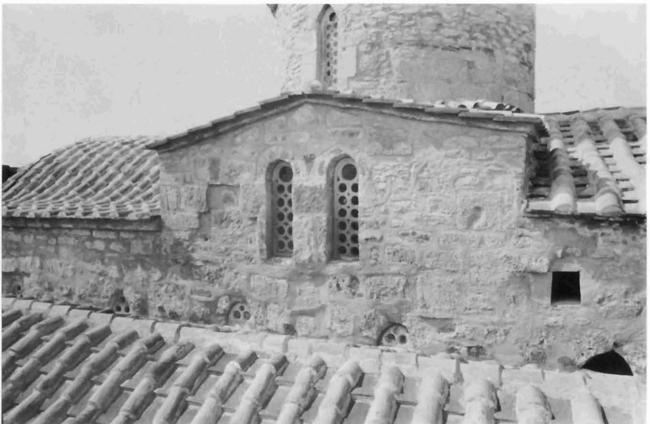
2. South Clerestory Windows
