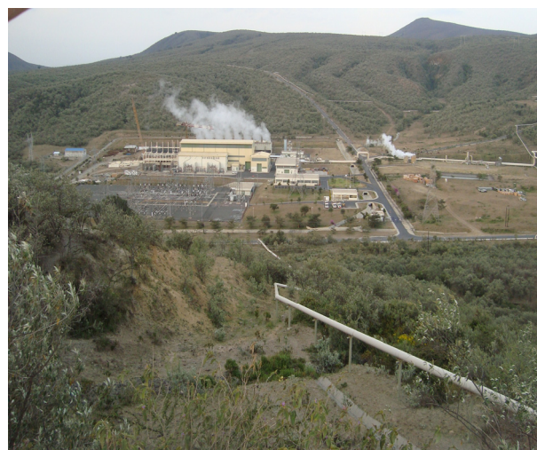
FIGURE 4: Olkaria II power station, Naivasha.
