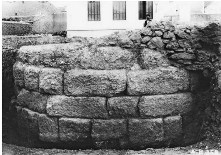
Figure 42. Remains of curtain wall behind the tower at Erysichthonos 20–24 (Th103) (at right and at far left). Photo courtesy Deutsches Archäologisches Institut (neg. D-DAI-ATH-Athen Bauten 361)
