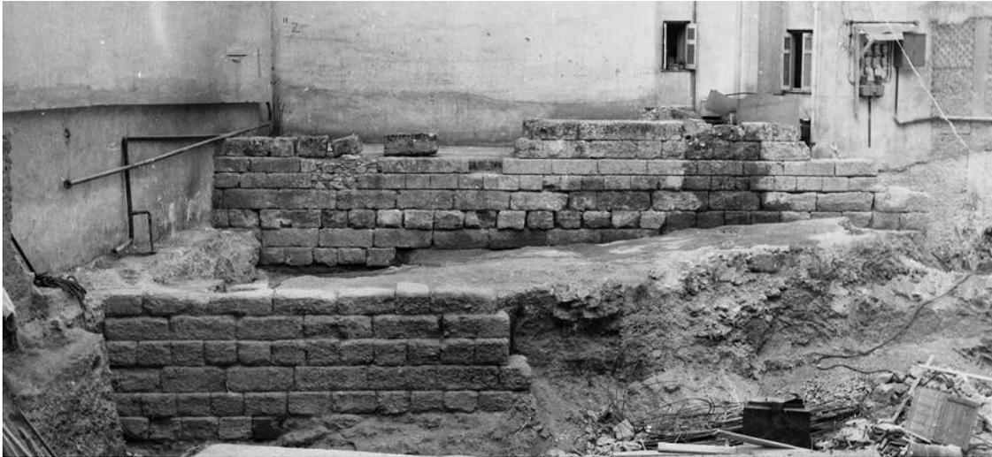
**Figure 31.** All-stone Hellenistic construction at the intersection of Aristeidou 14 and Pasmazoglou Street (Th29). Curtain wall at rear. External ring road (middle); *pro-teichisma* (foreground). Travlos Archive, photography folder 112 (Photographs from Athens). Courtesy Archaeological Society at Athens
