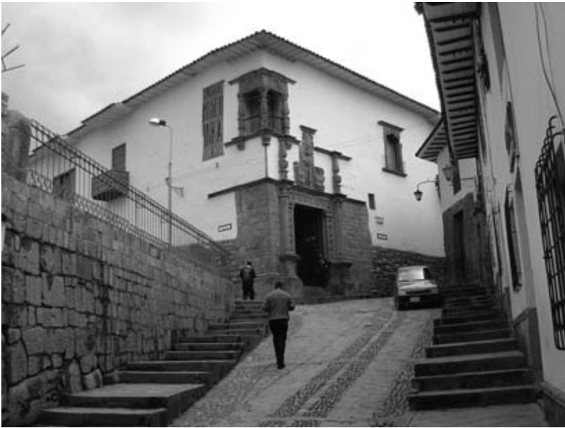
Figure 11.1 Looking up at the Museo Inka, Cusco, Peru. This Colonial Period building is known as the Casa del Almirante.
