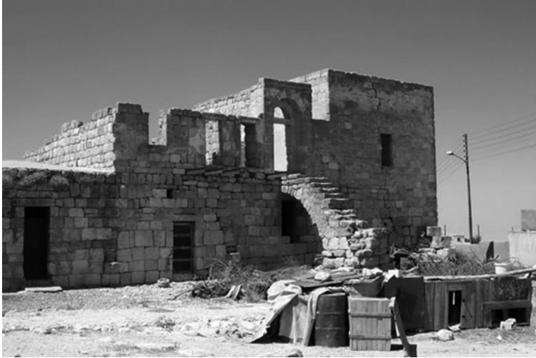
Fig. 5.3 The nineteenth-century farmhouse structure ( Beyt Nabulsi ) at Hisban. Domestic space, including a guesthouse, is located above storage rooms. (Courtesy of the author)
