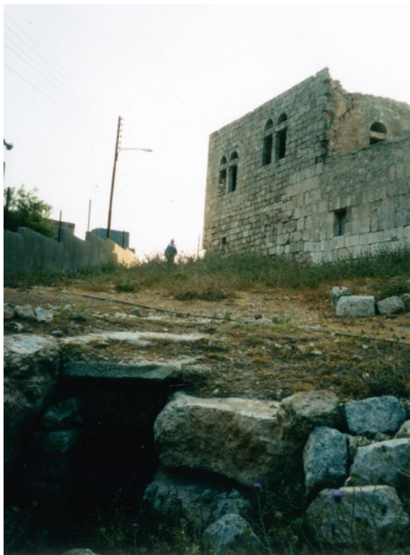
Fig. 5.5 Entrances to cave beneath Beyt Nabulsi (Courtesy of the author)
