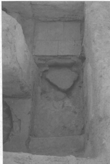
8. North-eastern branch of the sottoscala, view from the west
