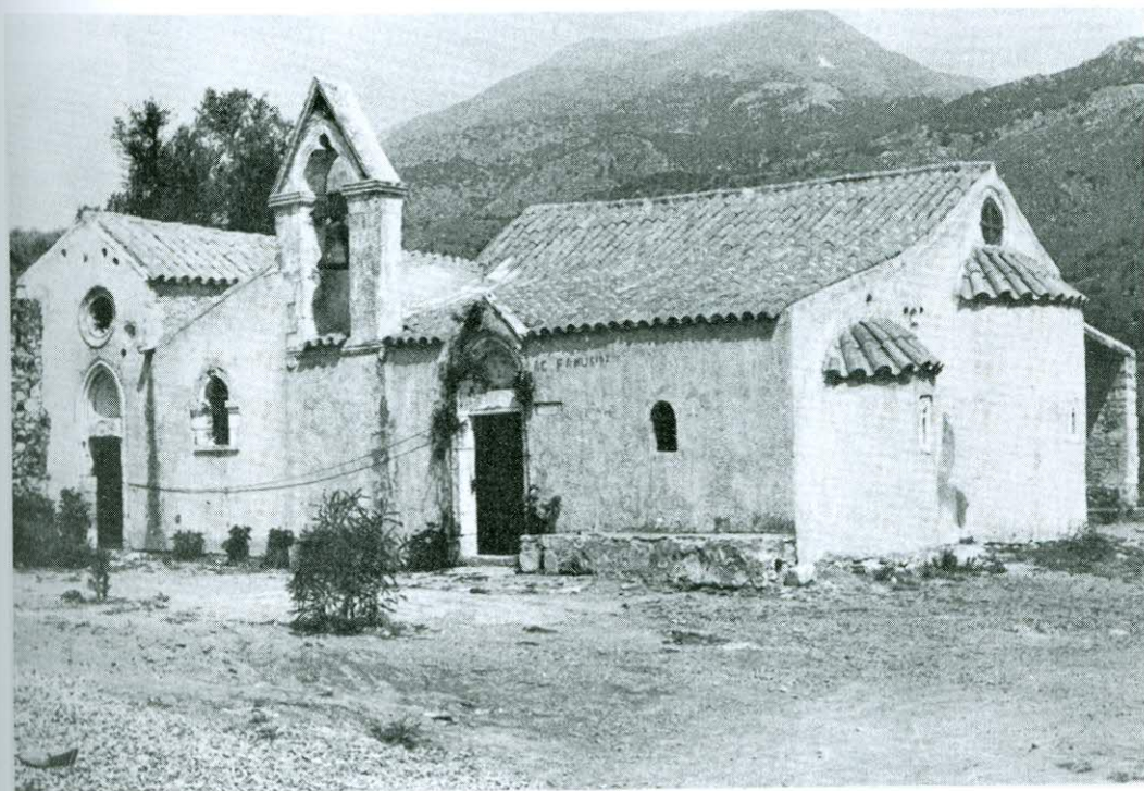
Fig. 5.3. Crete, Moni Varsamonerou. South-east façade.
