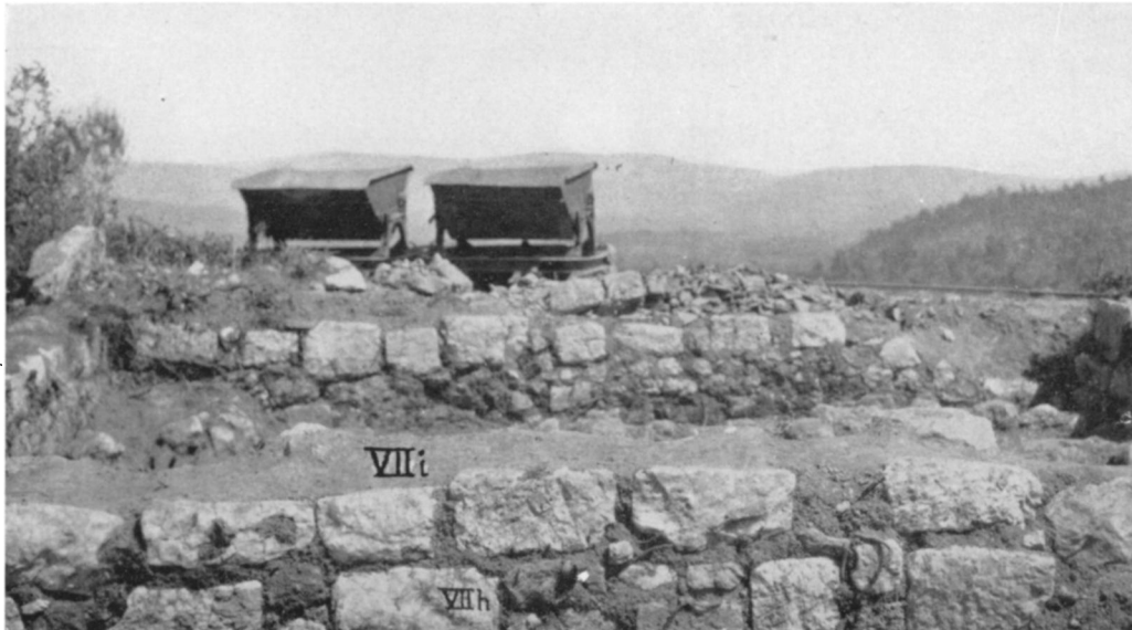
Fig. 12. Walls of Eastern Room in Western Section of North Wing of Stoa, Looking East Across Room
