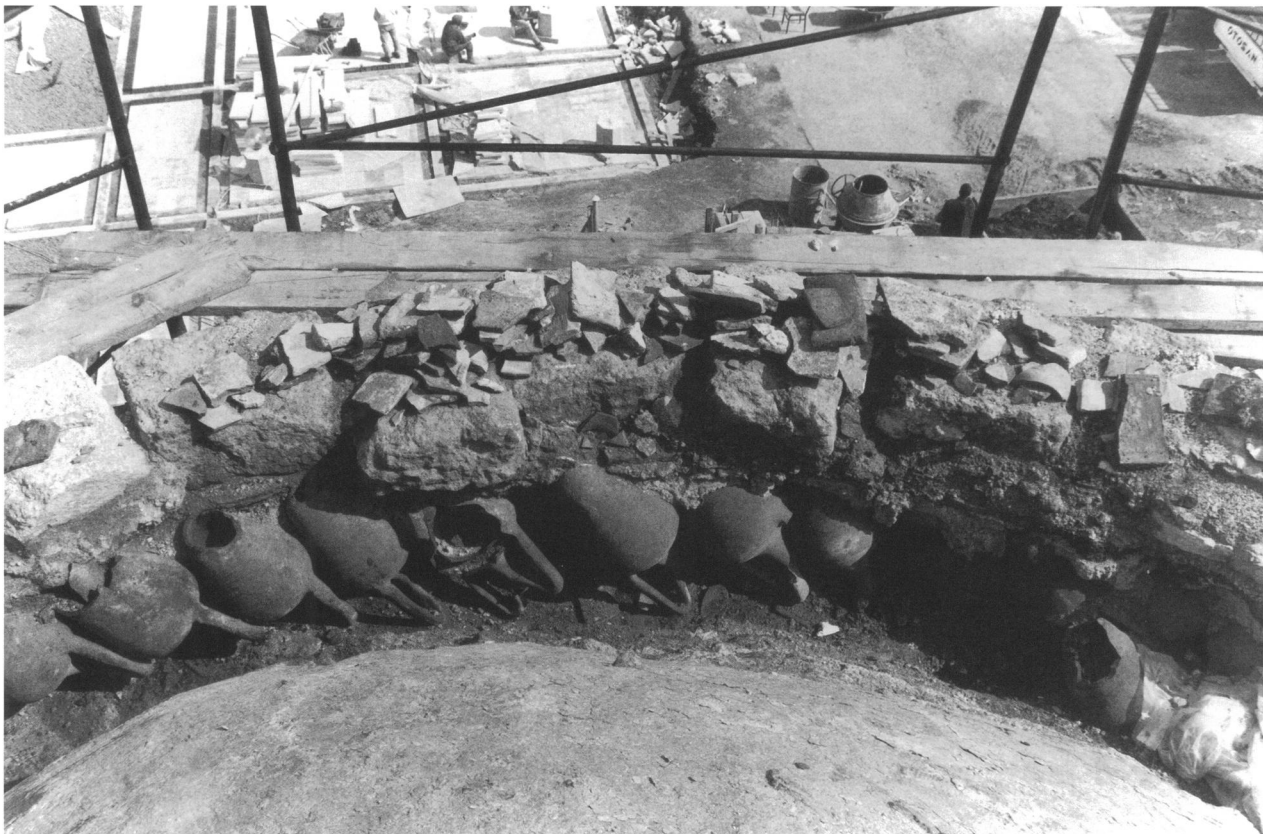
9 Zeyrek Camii, North Building, view toward the apse vault during cleaning, showing Byzantine amphorae in the fill behind the conch and Ottoman cornice blocks joined with iron ties, 1997
