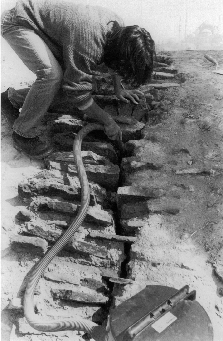
7 Zeyrek Camii, North Building, cleaning of crack in north crossarm, 1998
