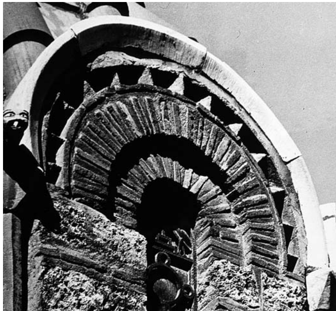
Fig. 5. Kapnikarea. The dome of the southern church
