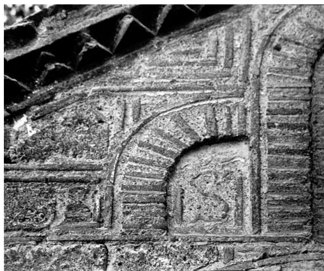
Fig. 11. Kapnikarea. Exonarthex, detail of masonry
