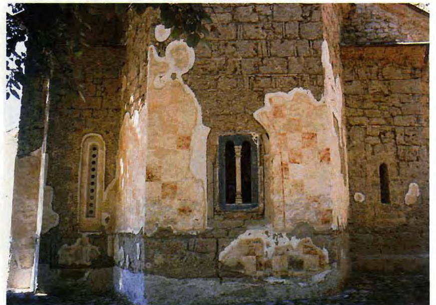
22. Banja. St. Nicholas; east facade showing painted 'building opus'.
