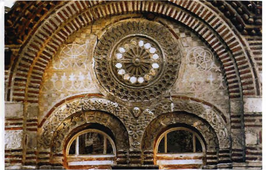
27. Hilandar Monastery. Katholikon, exonarthex; detail of north facade.
