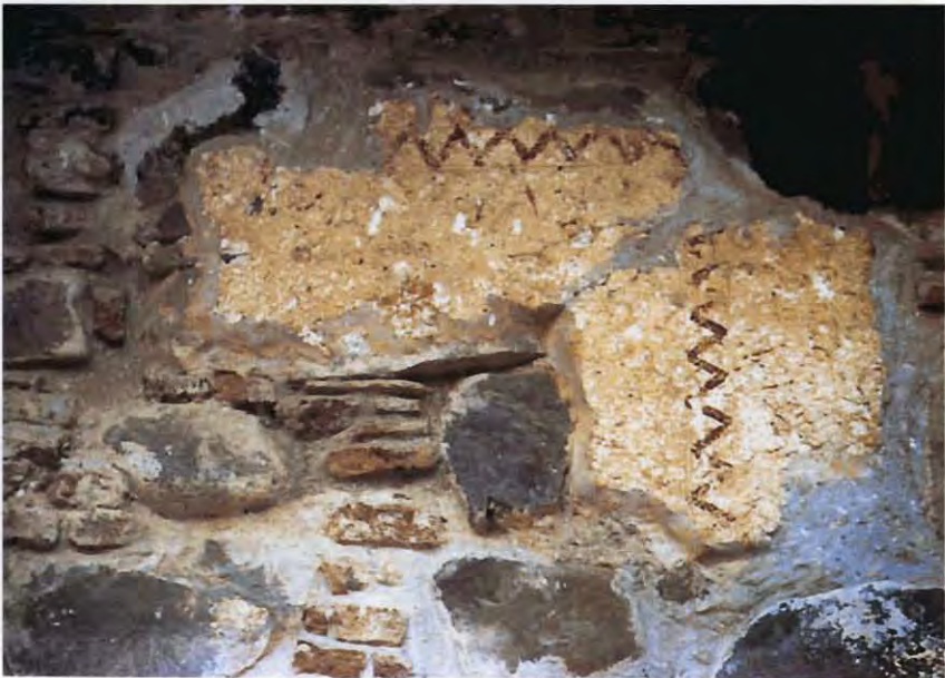
30. Asinou. Panagia Phorviotissa; south facade, detail of painted 'building opus'.
