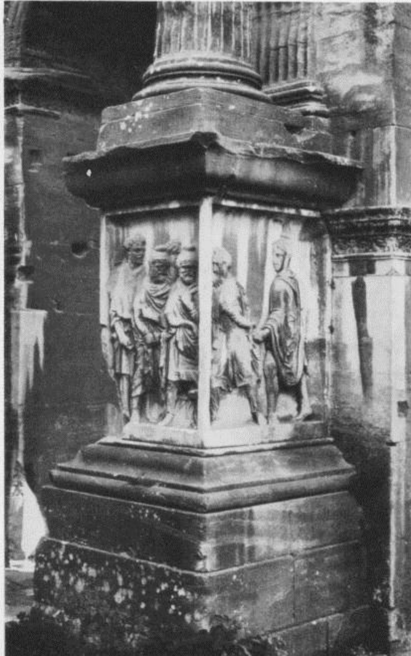
136 A pedestal from the west face on the left of the centre arch. GFN E/17543
