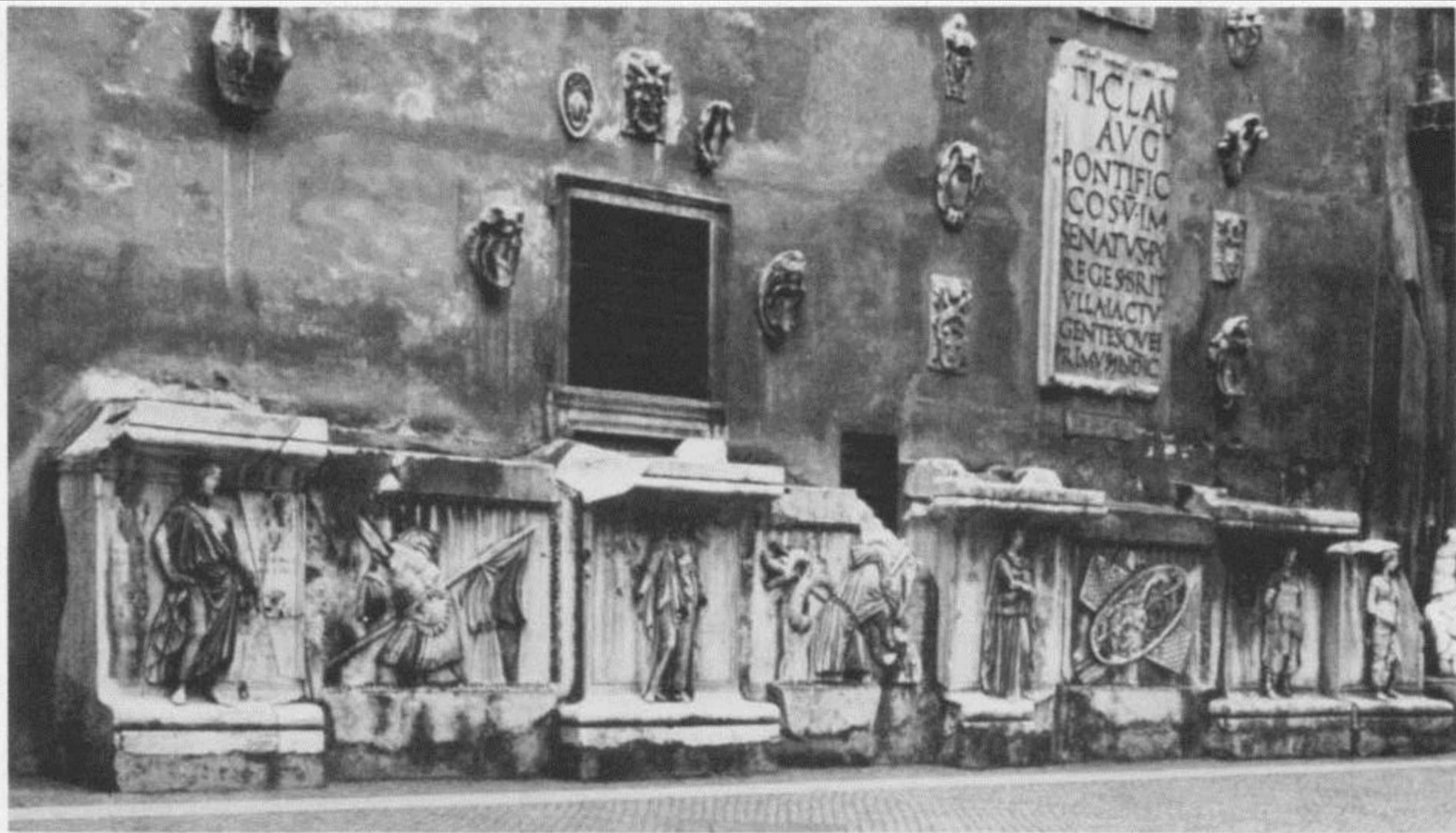
559 Marble balustrade composed of provinces and trophies collected in the courtyard of the Palazzo dei Conservatori.
