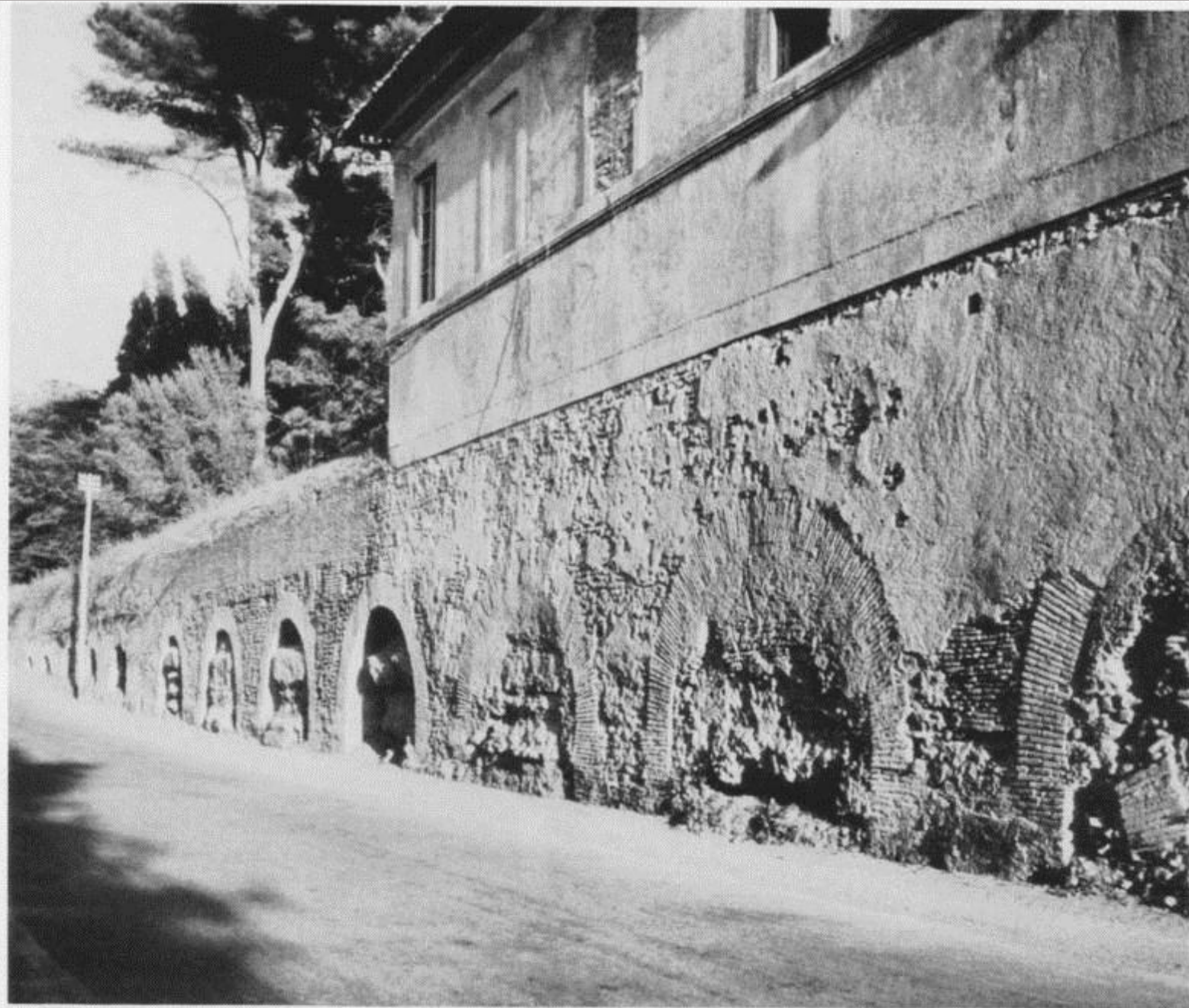
48 Arches of the Aqua Paola, a restoration of the Trajan aqueduct by Paul V in 1605, showing remains of the ancient arches and conduit.
