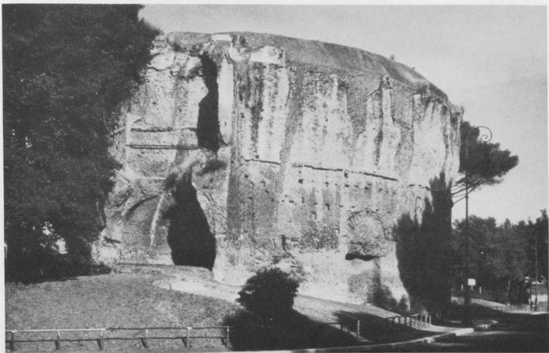
1289 Exterior, showing the corridor which lies behind the exedra; plan D.
