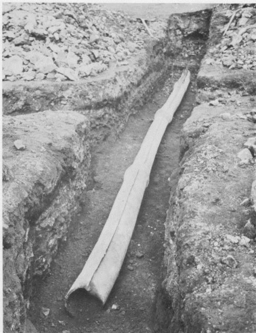
50 Part of an 18 m lead pipe found in situ within the Baths of Trajan. The part with the inscriptions is shown in fig. 49. Rip X C/3110
