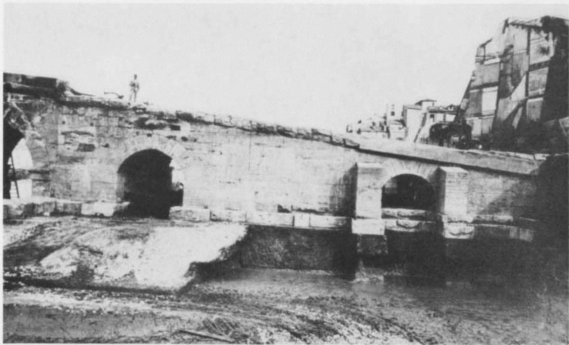
911 The ramp on the left bank of the Tiber seen from the south.
