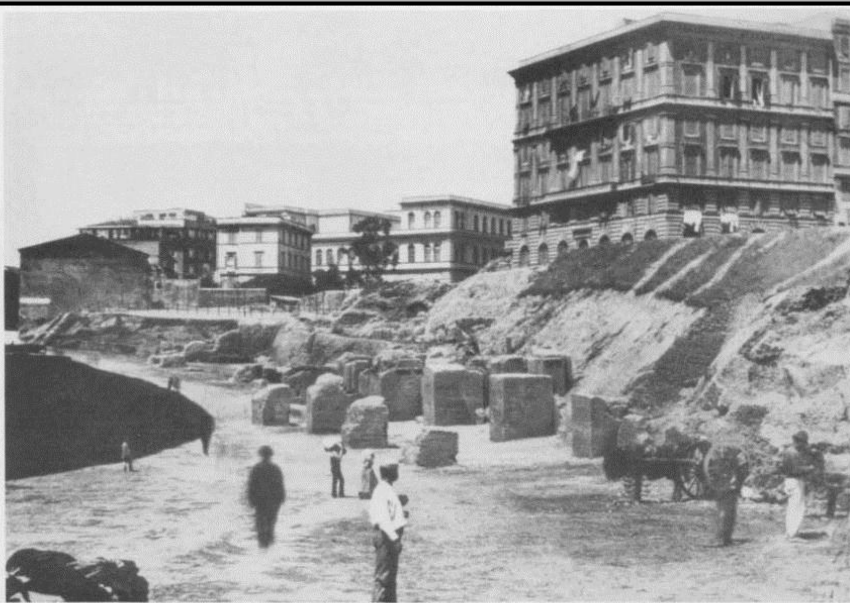
1282 The excavation of the porticus; the brick pilasters with half columns in the third row have survived, those in the front rows were destroyed.
