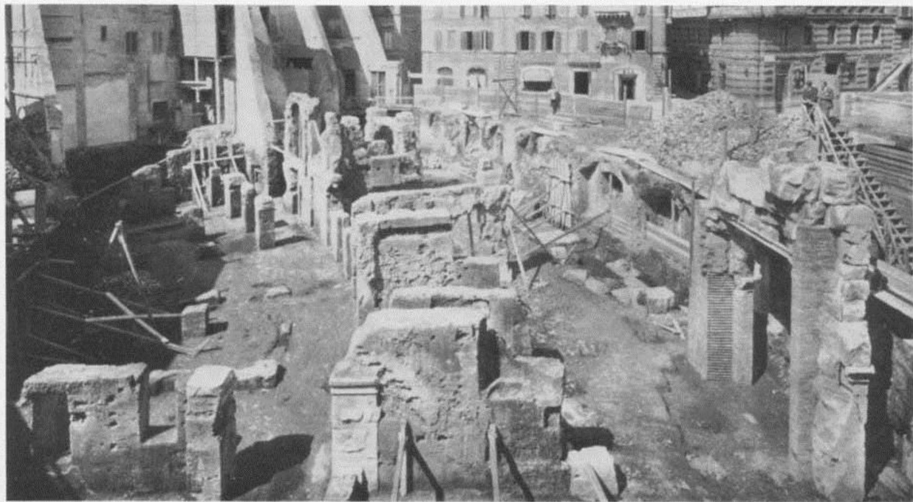
1177 Excavation of the north side of the stadium in 1936.
