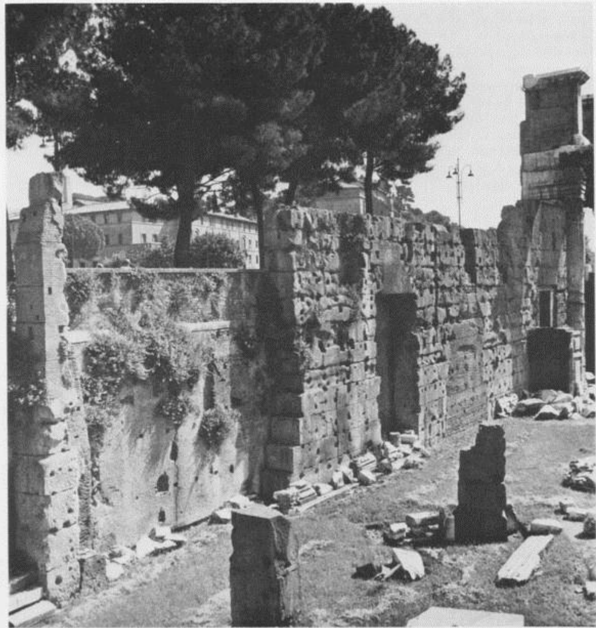
542 Part of the north-west perimeter wall of the Forum Pacis which is continued in the perimeter wall of the Forum of Nerva.
