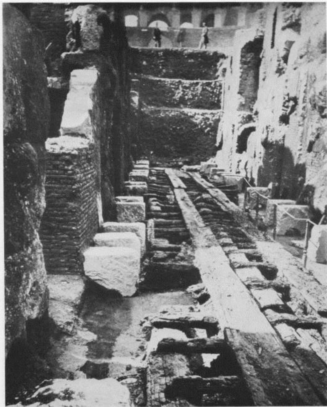
11 A wooden floor in the central gangway below the arena. It was discovered during the excavation of the foundations in 1875 and has since been lost.
