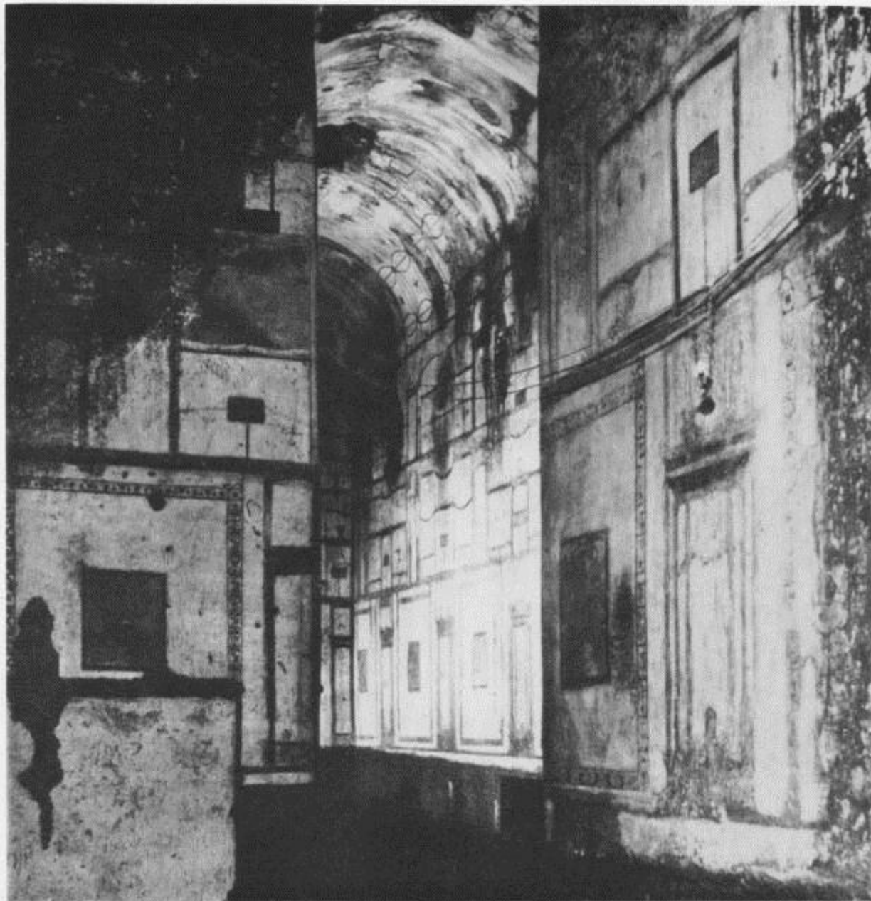
412 The corridor connecting the central block with the east wing (Plan No. 6).
