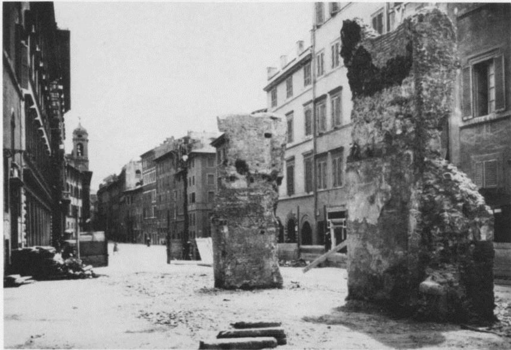
1268 Two brick piers, belonging to the western perimeter wall of the Baths of Nero, isolated and subsequently removed, during the construction of the Corso del Rinascimento.
