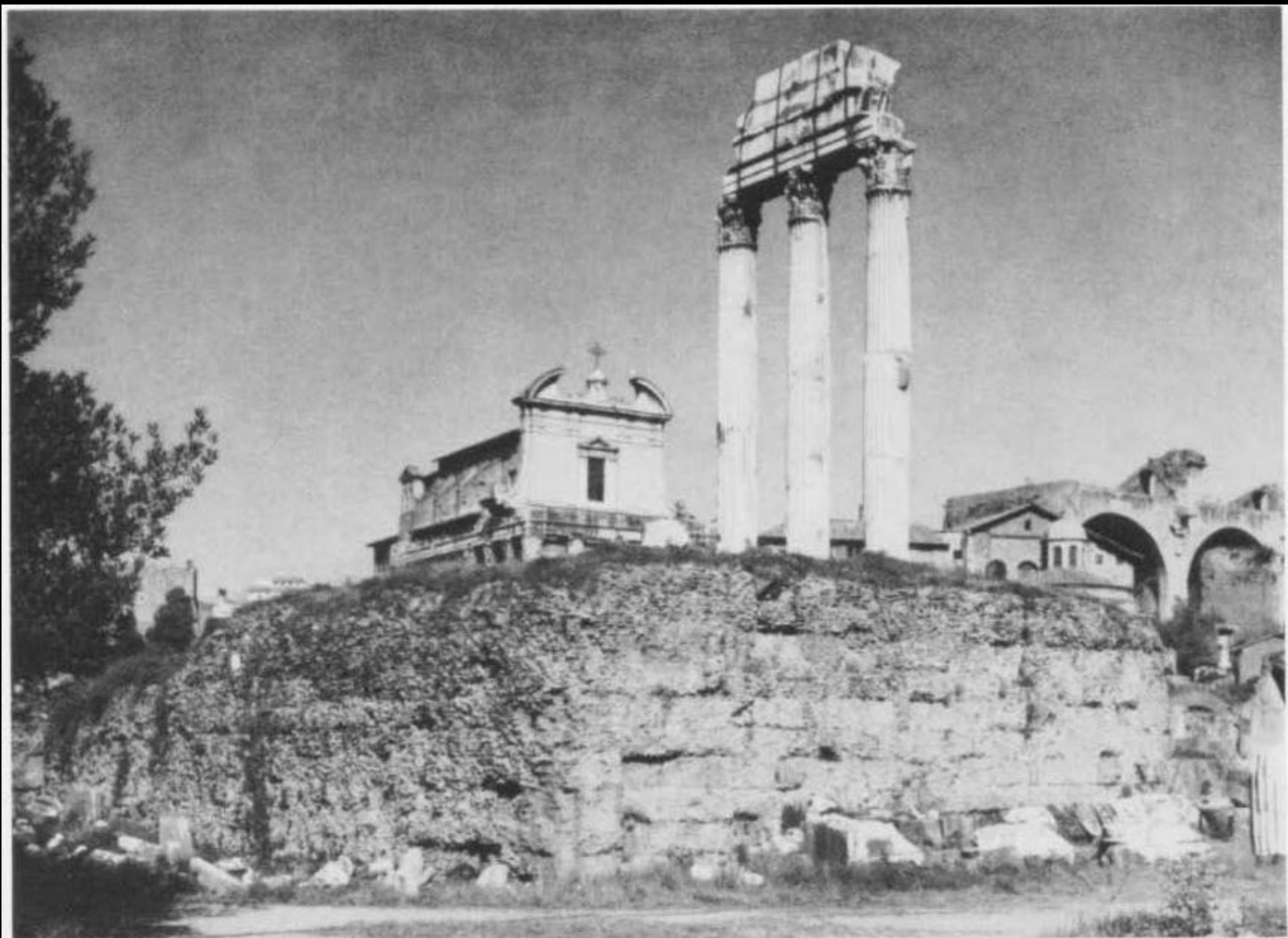
240 The core of the temple podium, south and west sides.
