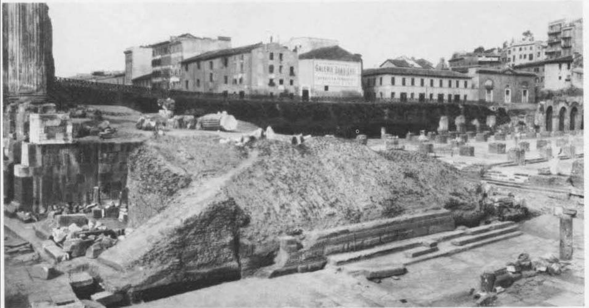
241 The front of the temple in 1895; no trace of the main stairway is seen; it was totally destroyed between 1871 and 1890. Inst Neg 714 B
