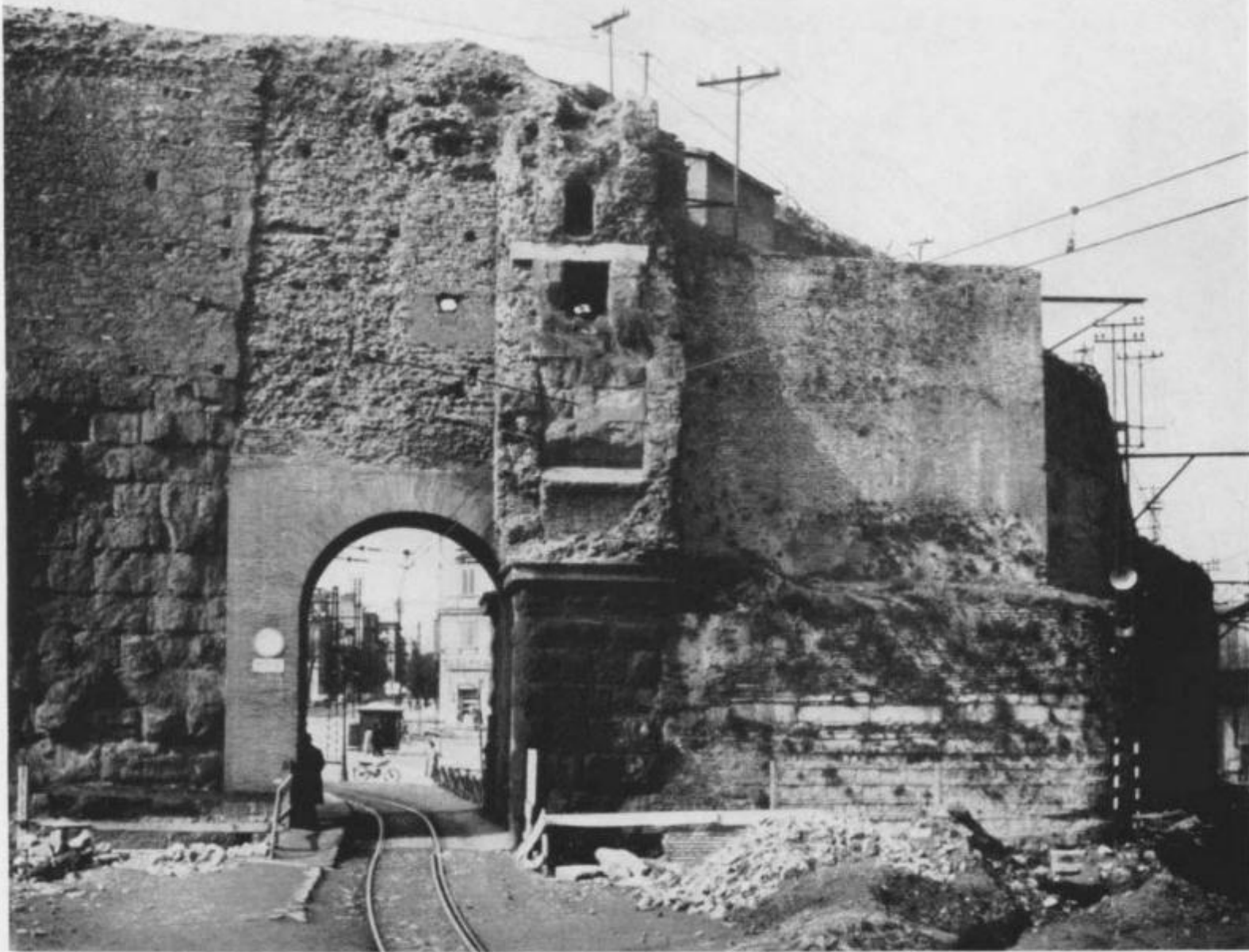
43 The conduits of the Aqua Marcia, Tepula and Iulia at the point where they pass through the Aurelian Wall, immediately to the north-east of Porta Maggiore. Fot 859
