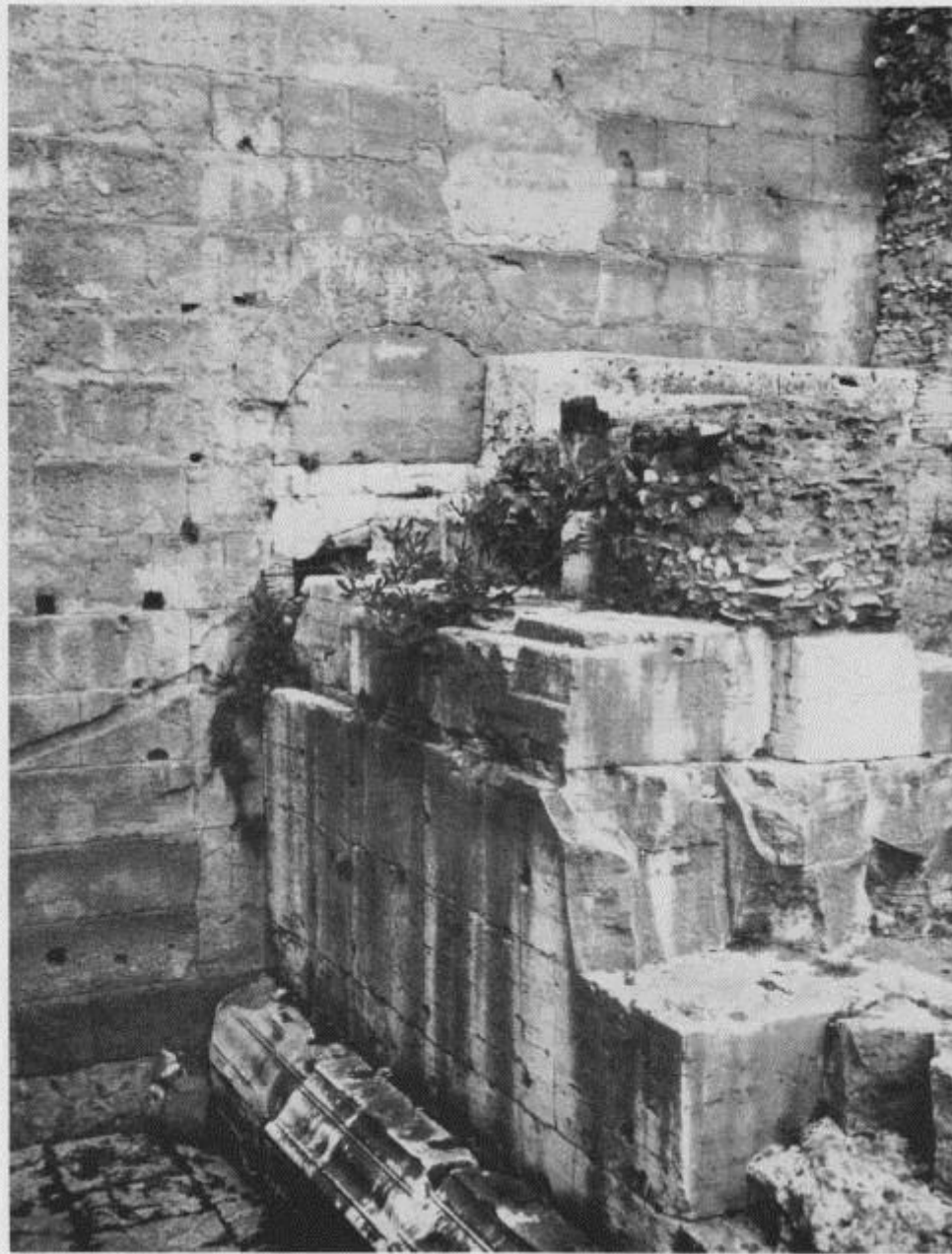
1197 The entrance from the Forum which was blocked by the podium of the Temple of Vespasian.
