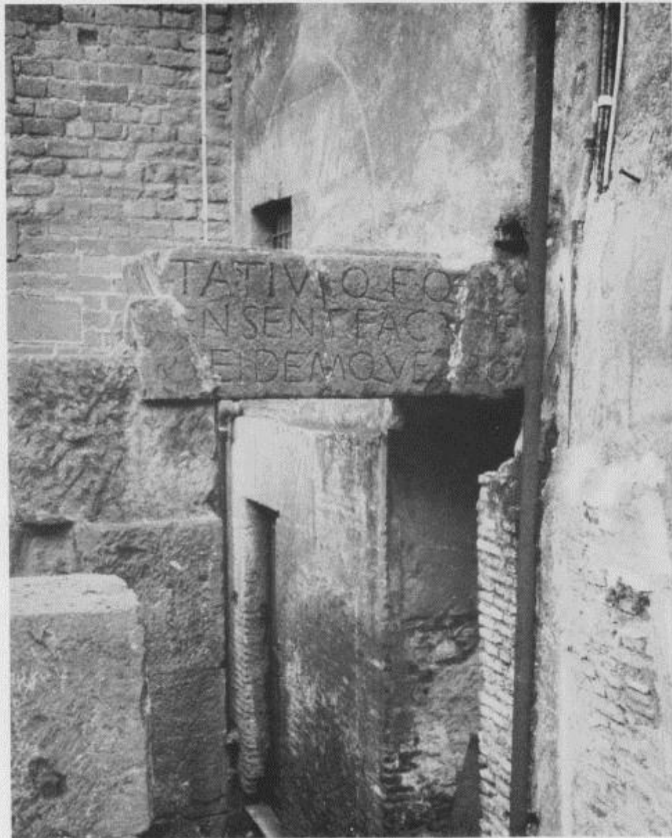
1199 The inscription of Lutatius Catulus (CIL VI, 1313) found inside the building by Canina in 1845, and set up on ancient door-posts on the northern outer wall. Fot 145
