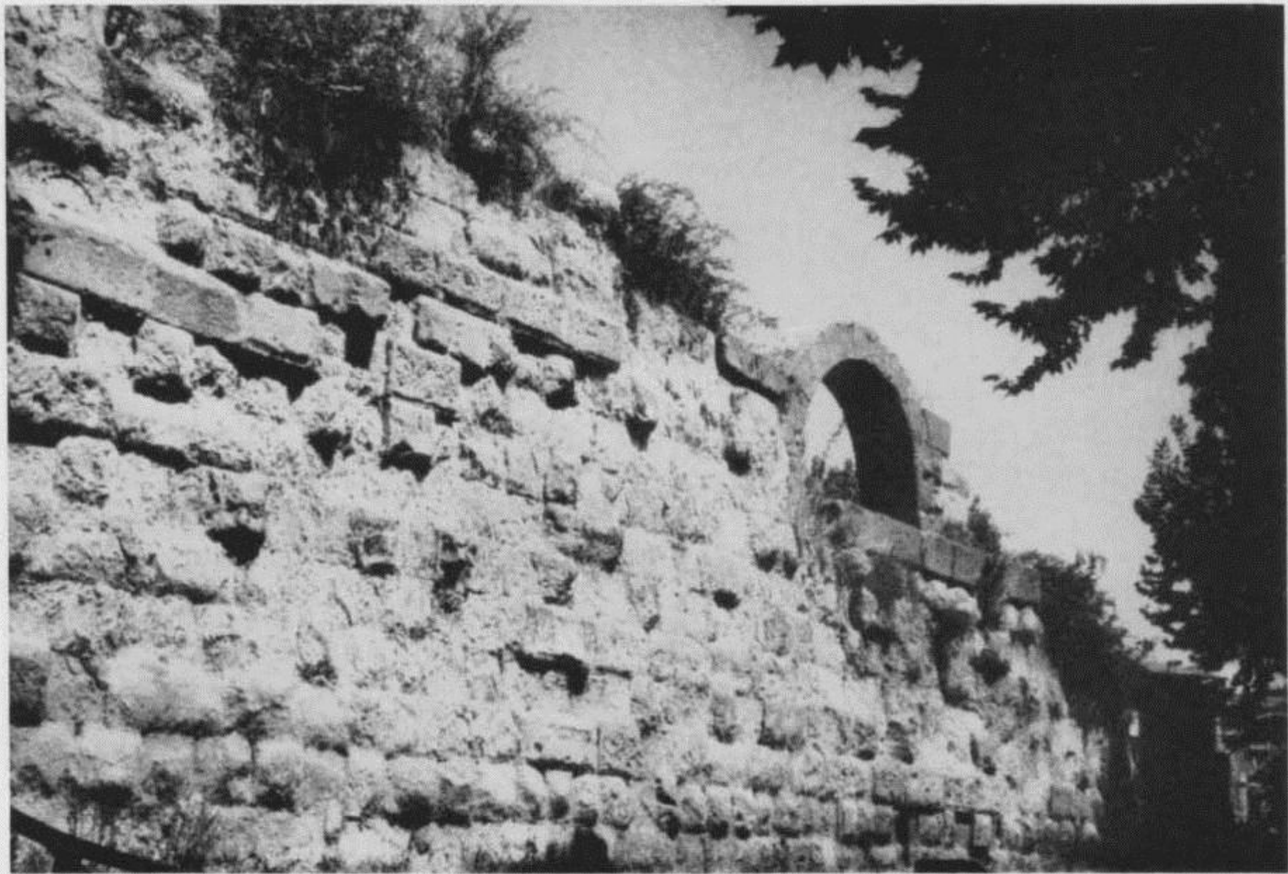
818 Outer view of the wall on the Aventine, showing an arched opening for a catapult.
