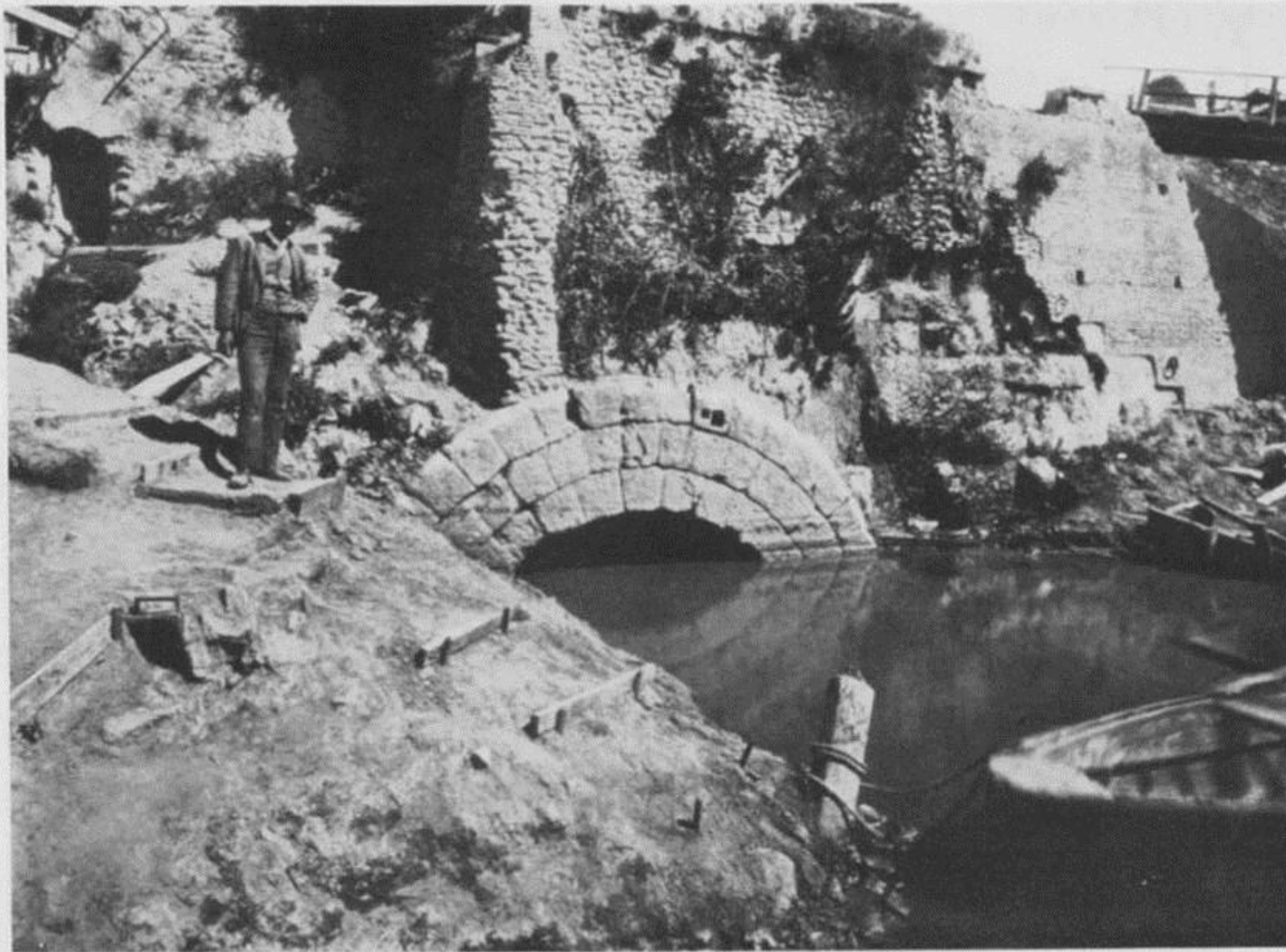
301 The mouth of the Cloaca Maxima in 1877, before the modern embankment was built.
