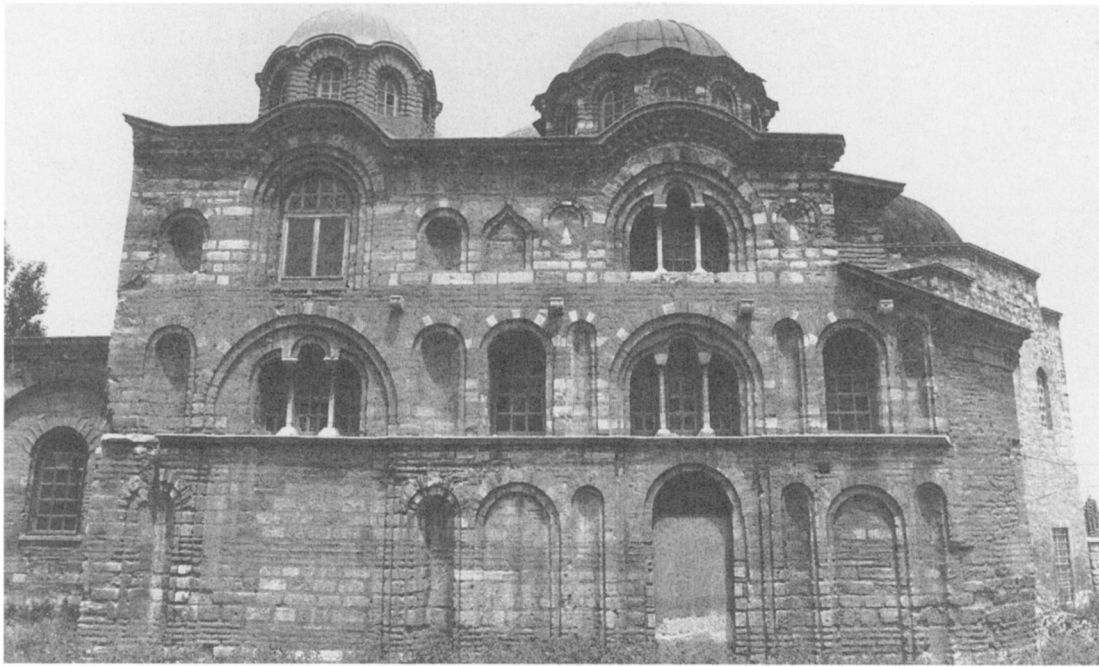
FIGURE 10. Constantinople, Pammakaristos church (Fethiye Camii), south facade of the parekklesion (photo: author).
