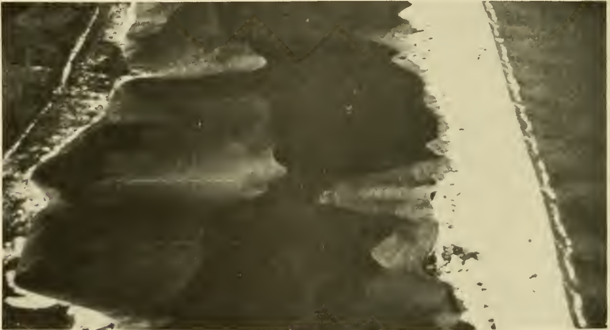
Figure 1-4. Undeveloped barrier island on the gulf coast of Alabama after Hurricane Frederic.
