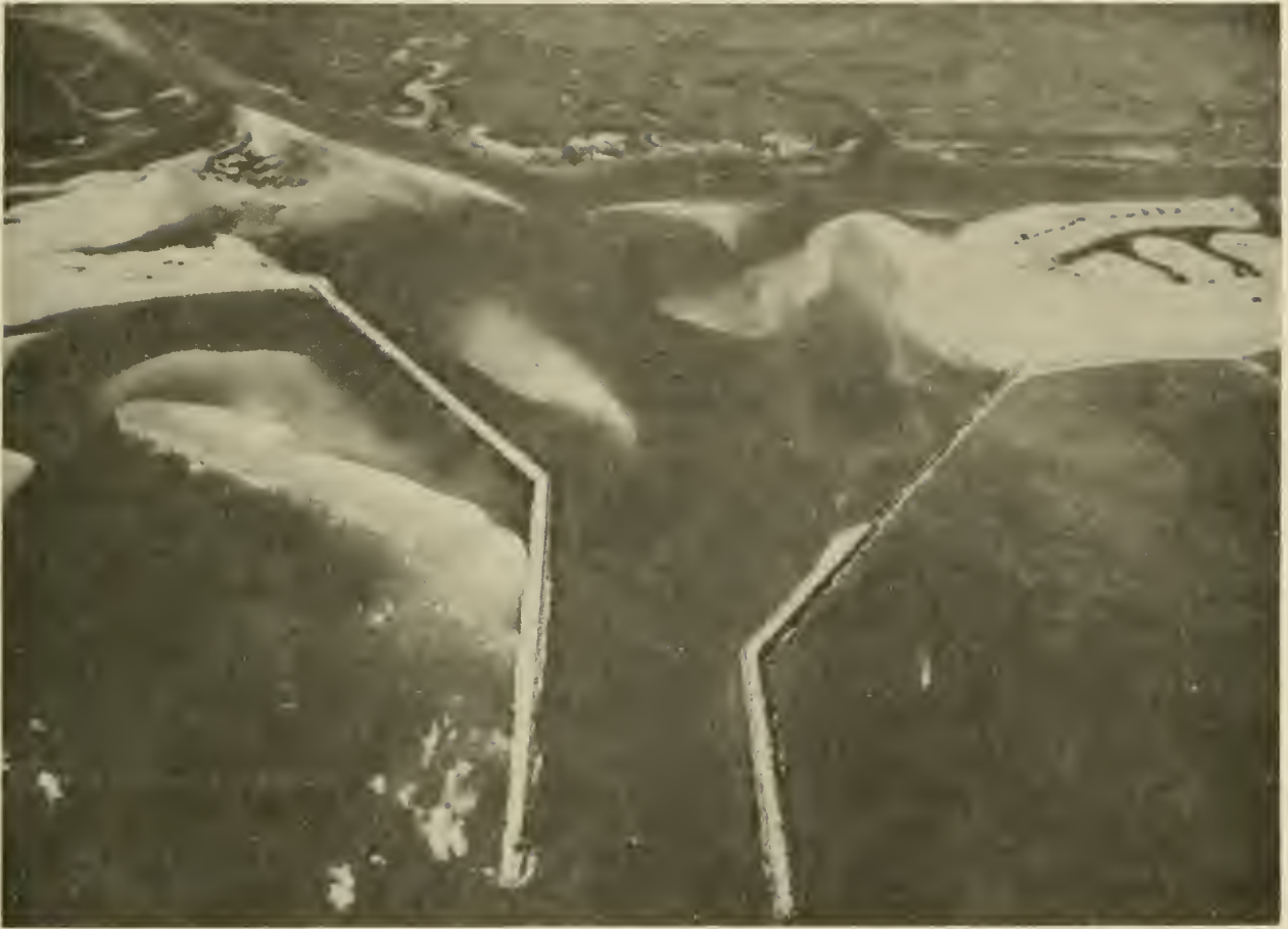
Figure 1-13. Weir jetty at Murrells Inlet, South Carolina, 1981.
