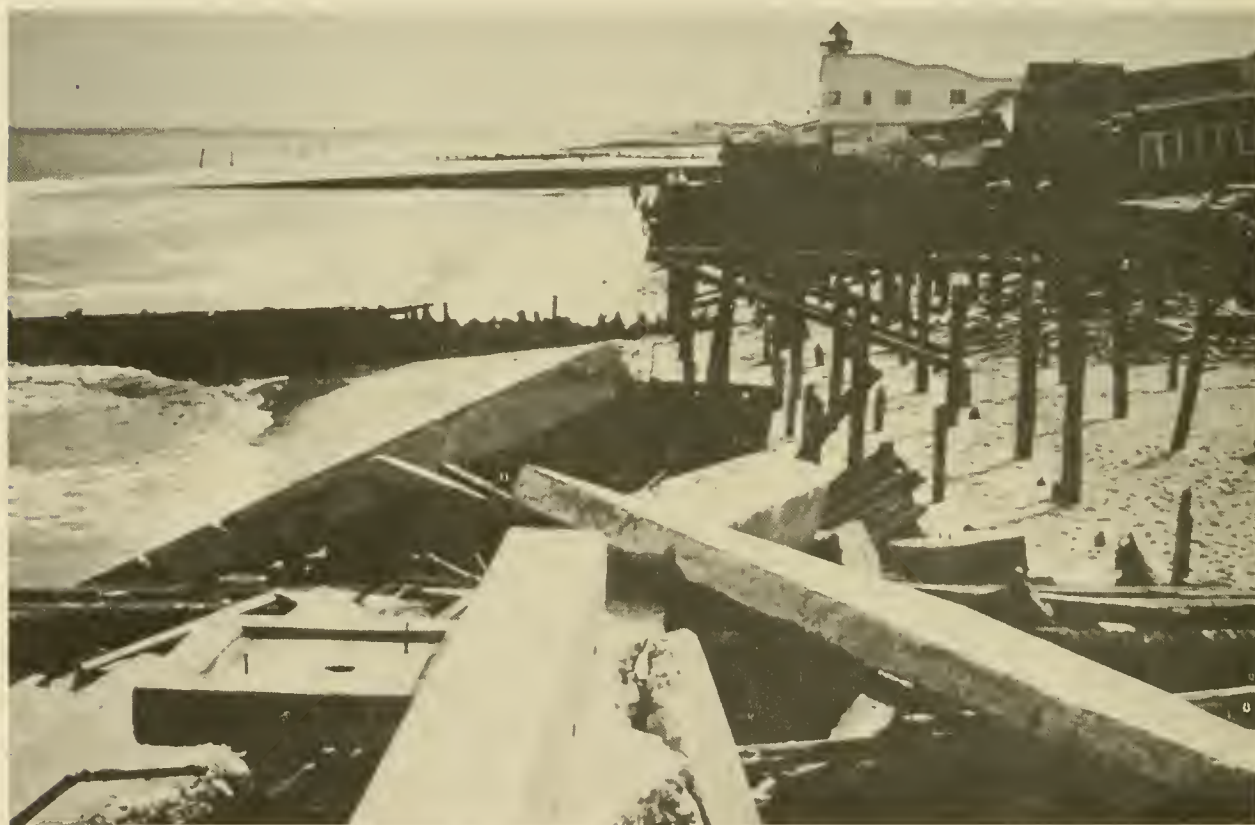
Figure 1-10. Damage after the 1962 storm, Rehoboth Beach, Delaware.
