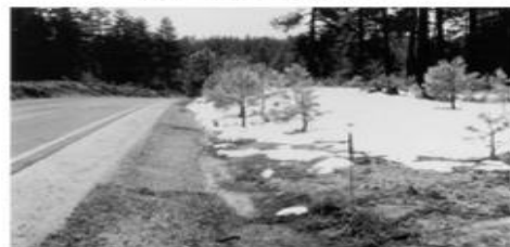
Typical Roadway with Roadside Hazard Rating Equal to 3.
