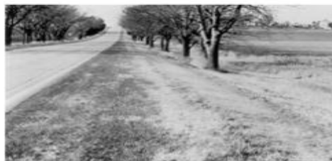
Typical Roadway with Roadside Hazard Rating Equal to 5.
