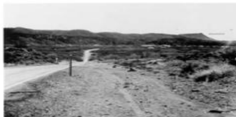
Typical Roadway with Roadside Hazard Rating Equal to 2.
