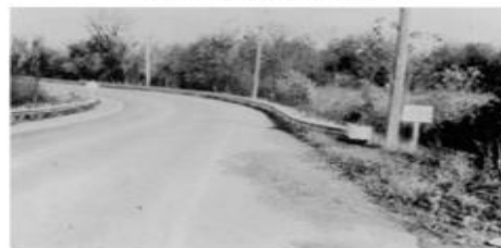
Typical Roadway with Roadside Hazard Rating Equal to 4.
