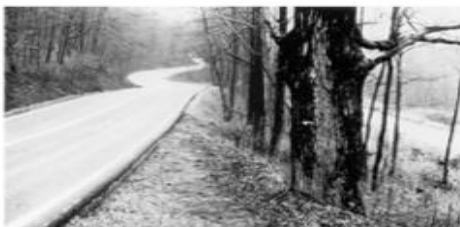
Typical Roadway with Roadside Hazard Rating Equal to 6.
