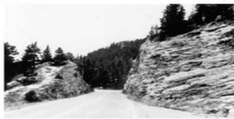
Typical Roadway with Roadside Hazard Rating Equal to 7.
