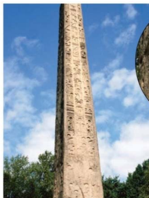
(b) After acid rain damage
