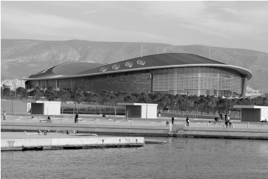
Figure 11.4: Faliró Bay Complex.
